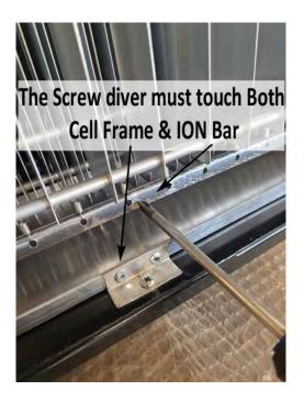
Remove the ground screw. The ground screw secures the filter cell and provides the ground needed to allow the filter cell to function properly
