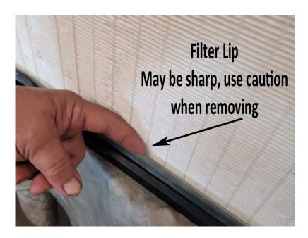
Move the filter back and forth with a side-to-side motion drawing it slowly to you. You can reinstall the filter in the same manner gently moving the filter back into place. The main filter should touch the carbon filter.
