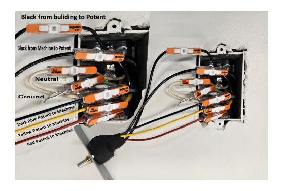
You do not have to use the LakeAir Wiring Kit, Low voltage speed control is often hooked up using thermostat wire. Be sure to use a heavy enough gauge wire for the air purifier (maximum 4.4 amps per unit)
